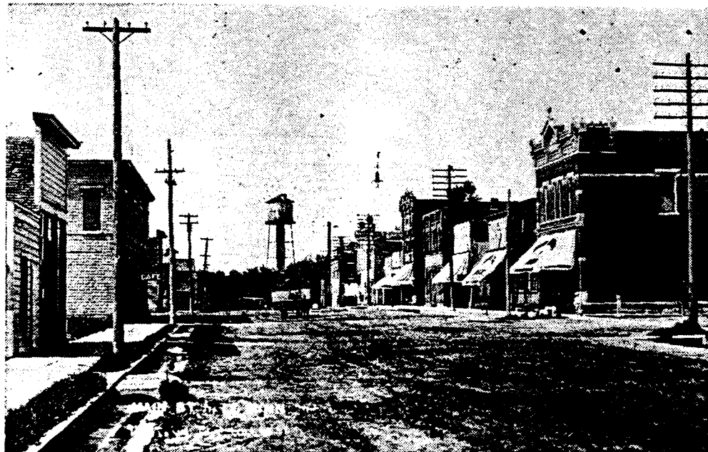
Main street looking north. Before autos came to Lyle. The smoke stack near the water tower is part of building that housed Lyle's Power Plant.
