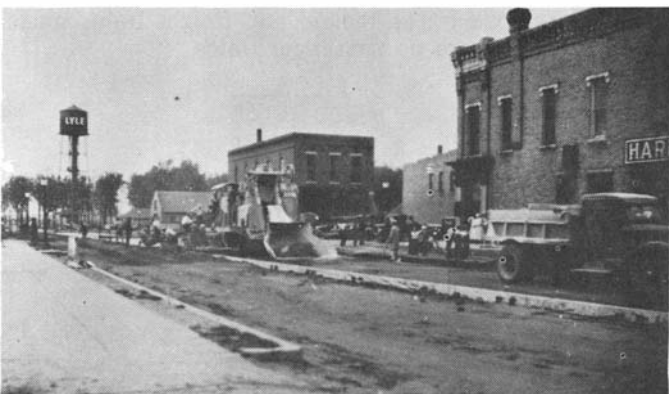
PAVING OF MAIN STREET
