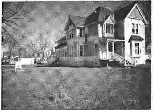
Beverly Frank's Bridal Shop, basement of old "Mortenson" home, Gingerbread trim, renovated by them, for business and home use.
