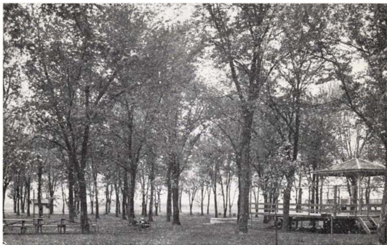
Later Park Photo. Platform on wheels used for street concert.
